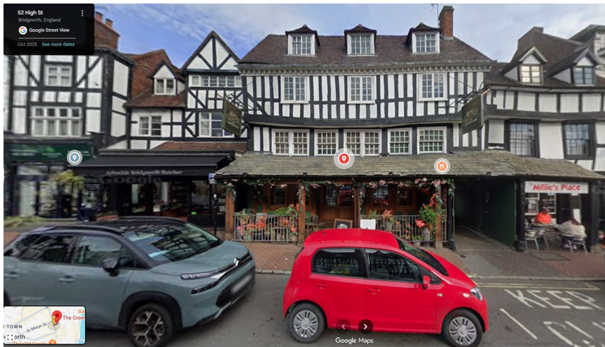
Facing the premises from High Street
